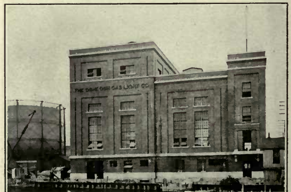
New Electric Plant of Oshkosh Gas Company, Oshkosh, Wis. Wm. A. Baehr, Chief Consulting and Constructing Engineer
